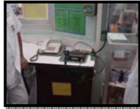
Radio Center, Community Hospital
